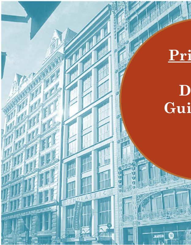
The Scholastic Building was the first new building to be constructed in the SoHo Cast Iron Historic District in New York City. The building's columnar Broadway façade complements the character of its neighboring cast iron buildings through the use of quality, long-lasting materials including steel, terracotta, and stone. While it echoes the scale and rich, formal character of the historic buildings in the District, it also illustrates how new designs can relate to historic styles while being clearly modern
