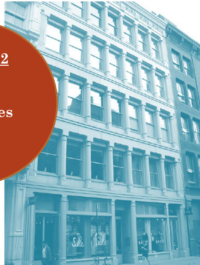
This building on Greene Street in SoHo shows how the cast iron kit-of-parts can be reinterpreted for infill construction in a crisp, modern manner. It was designed in pressed enameled steel, reflecting the technology of the 20th century in a 19th-century context.
