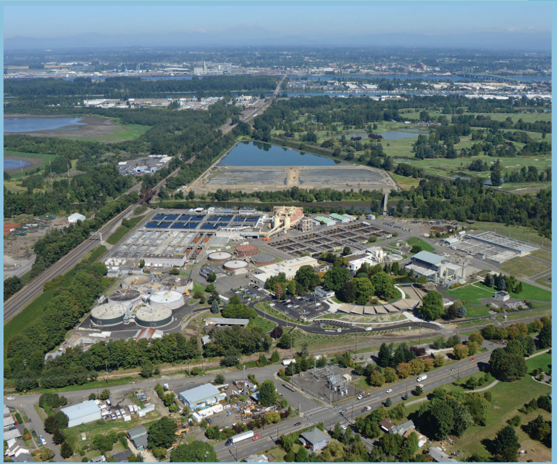
The Columbia Boulevard Wastewater Treatment Plant in North Portland
