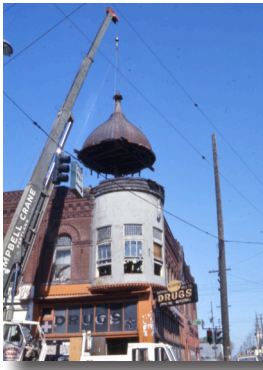
Removal of the Cupola on N Russell and N Williams for the Emanuel Hospital urban renewal area, 1973. A2010-003
