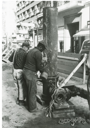
Sewer construction on SW 5th and SW Alder with workers, 1955.
