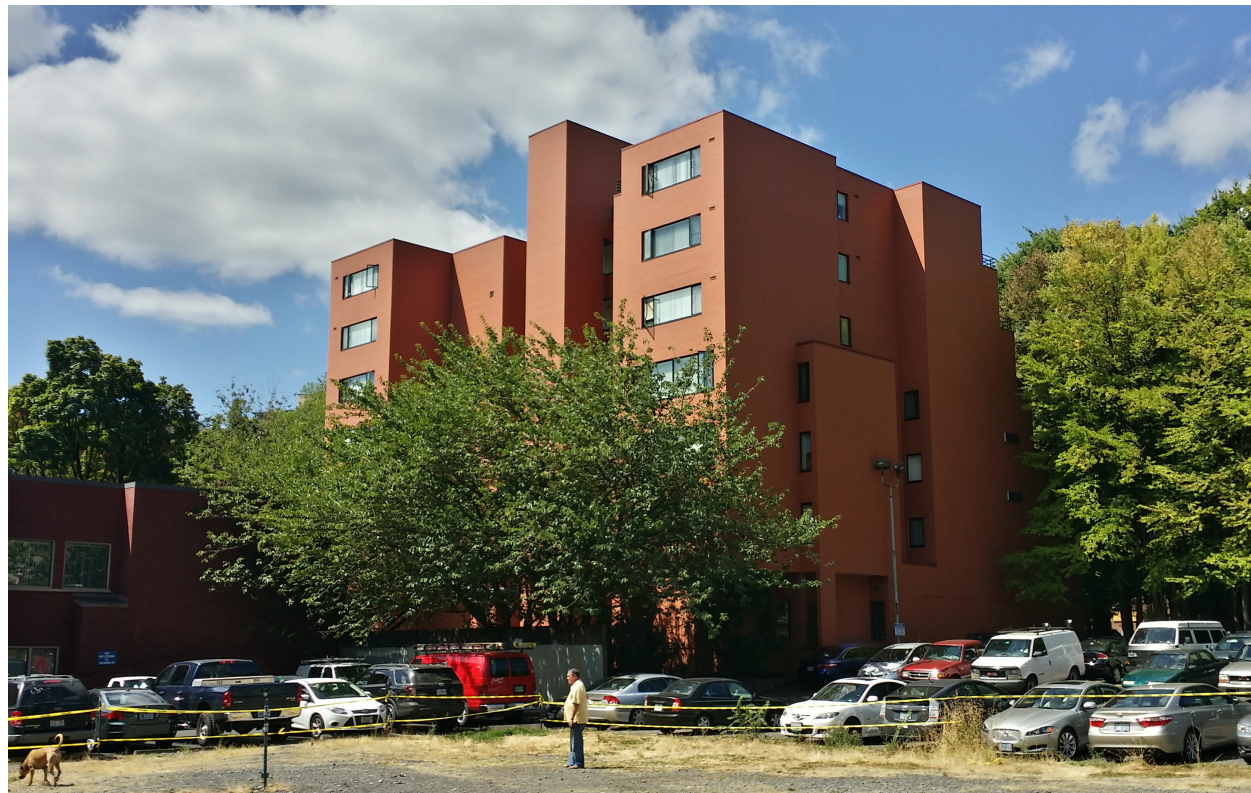
VIEW ACROSS SITE TOWARDS THE NEIGHBORING 1/4 EXISTING BUILDING
