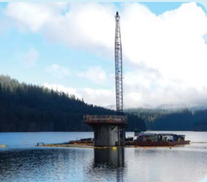
Construction at Dam 2 tower
