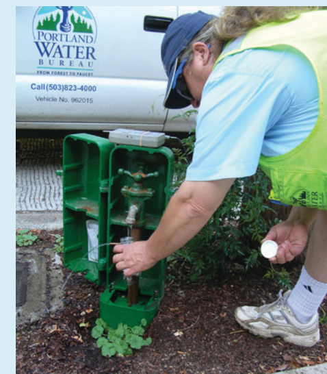
The Portland Water Bureau has 184 water quality sampling stations throughout the distribution system to monitor water quality on a regular basis.
