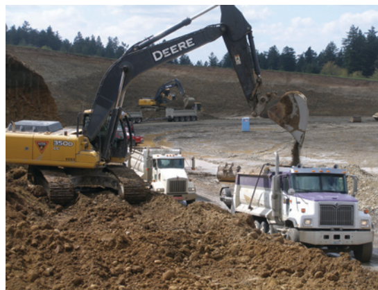
Excavation for the Powell Butte storage reservoir
