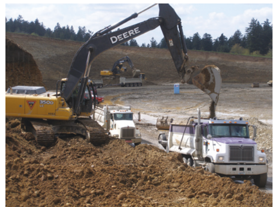
Excavation for the Powell Butte storage reservoir
