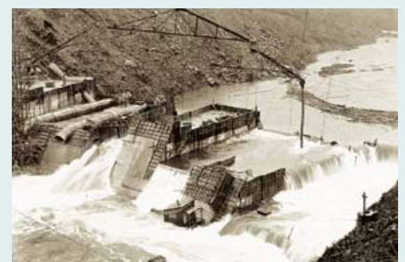
Eighty years ago construction of the first dam in the Bull Run was completed. Dam One, a concrete gravity arch dam, took two years to build, is 200 feet high and created a reservoir capable of storing approximately 10 billion gallons of drinking water.
