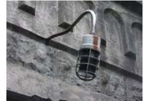
Historic exterior light over door
