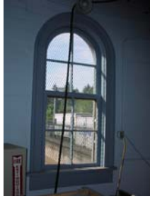
Typical Window, Gatehouse 5
