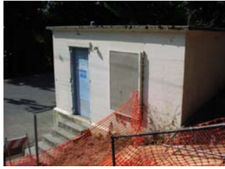
44" Meter House Reservoir 1
