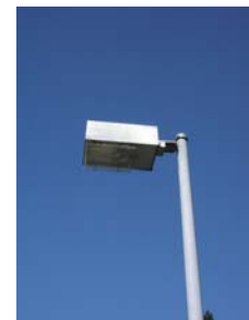
Non-historic light posts, Reservoir 5
