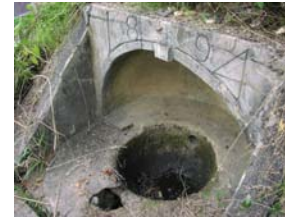
Reservoir 1 Fountain Structure
