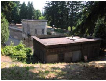
Reservoir 1 Weir Building
