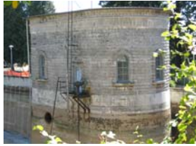
Metal Balcony, Gatehouse 1
