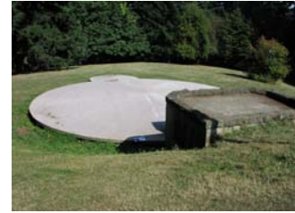
Reservoir 7 Underground Tank Structure
