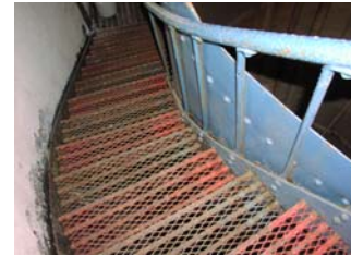
Curved iron stairway, interior Gatehouse 1
