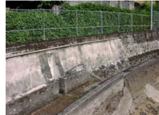
Reservoir Structure, Reservoir 1
