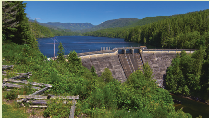
Dam 1 in the Bull Run watershed
