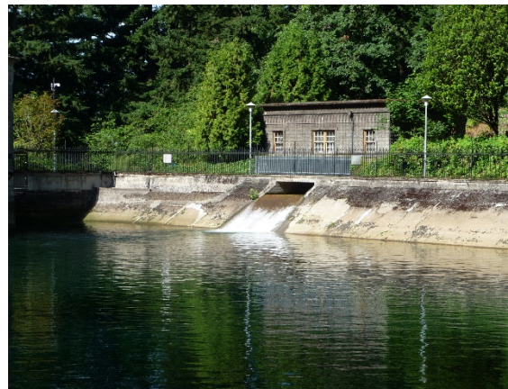
Figure 33. Reservoir 1 weir opening to be screened
