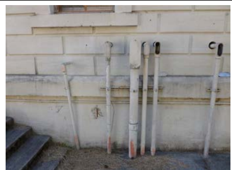
Figure 48. Gatehouse 6 East showing existing wall penetrations and conduits. Front view.
