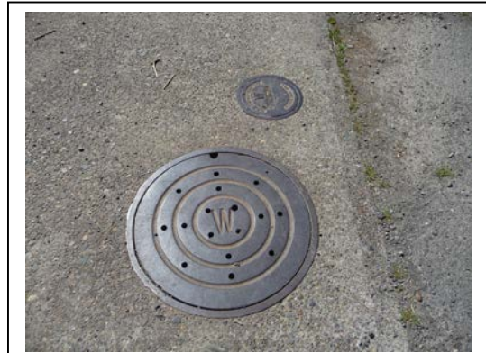
Figure 13. Manhole and CIV in road on Lincoln Drive
