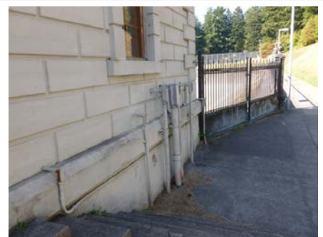
Figure 47. Gatehouse 6 East showing existing penetrations with condulets and conduits. Side view.
