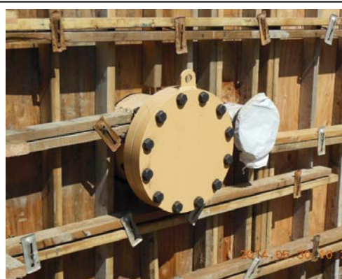
Figure 37. Typical blind flange (or cap).
