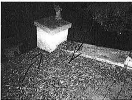
Front porch debris: Vertical wall joints will need patching at this point:
