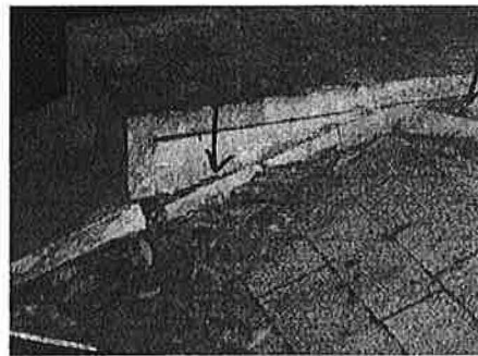
Front porch debris: Vertical wall joints will need patching at this point:
