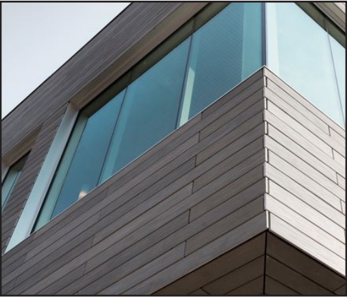
REPRESENTATIVE IMAGE OF VARIEGATED GFRC PLANKS. TO BE USED AT BALCONIES, RETAIL ENTRANCES AND LOBBY CEILING. COLOR AS SHOWN ON MATERIALS PAGE.
