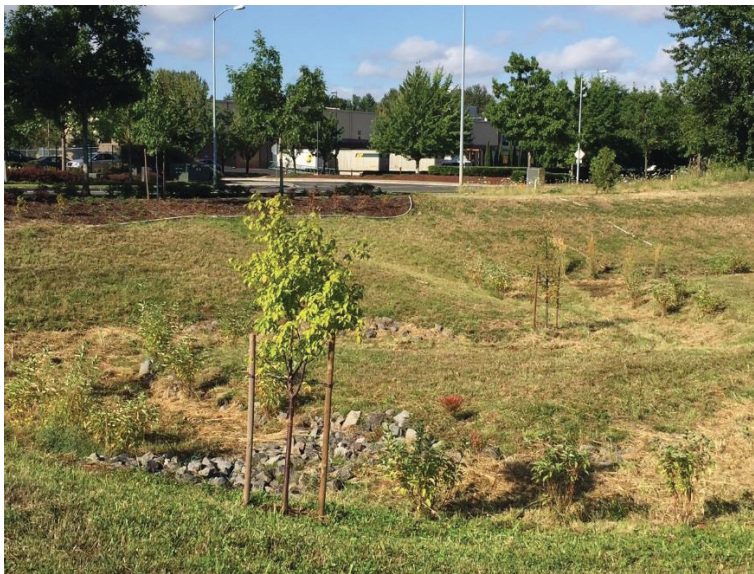
Wide swales, native landscaping, and downward-shining exterior lighting can improve stormwater and habitat functions, like shown here on industrial sites near PDX Airport.
