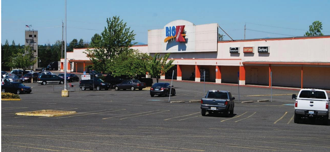
EG2 General Employment zoning is proposed at the Kmart/Sears site at NE 122 nd and Sandy.
