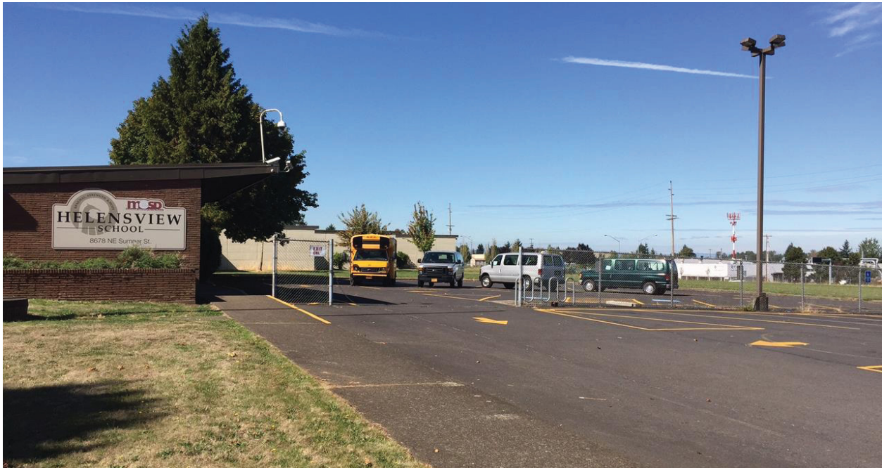
EG1 General Employment zoning is proposed at Helensview High School on NE Killingsworth.
