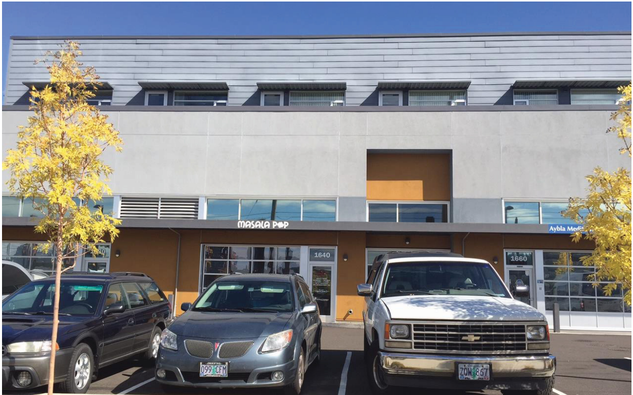
Code changes to allow Industrial Office uses are proposed in all IG1 zones in the Central Eastside, including the new construction sites at SE 3 rd and Clay shown here.
