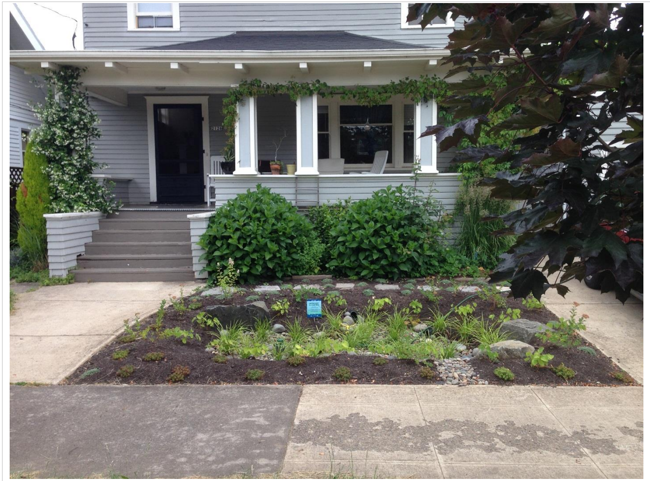
Figure 5-2 Example rain garden, installed in FY 2014
