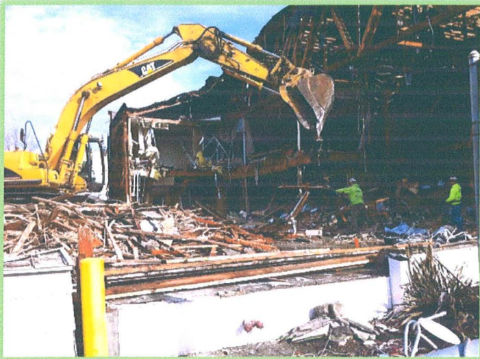
Demolition Mechanical removal
