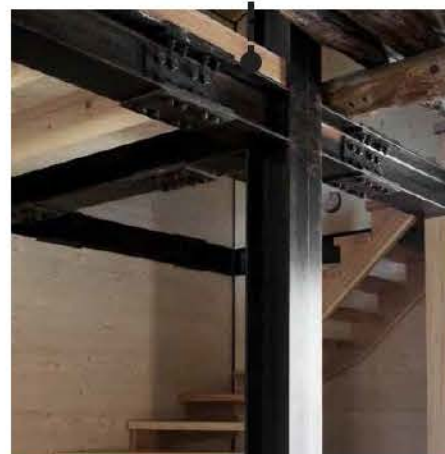
Painted steel structure
