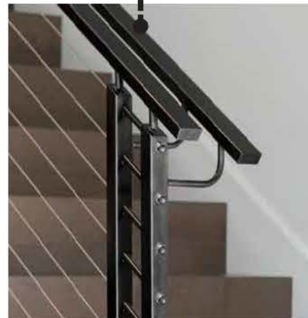
Painted steel flange-t-bar rails w/ SST cables
