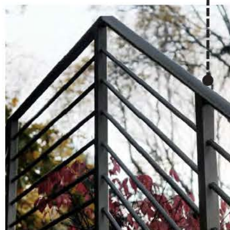
Painted steel rails w/ horiz. rods
