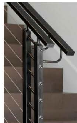
Painted steel rails w/ SST cables
