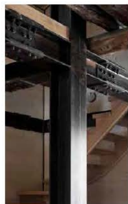
Painted steel structure
