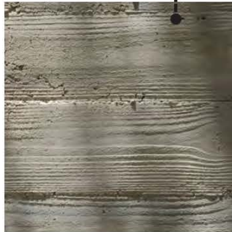
Board - Formed Concrete
