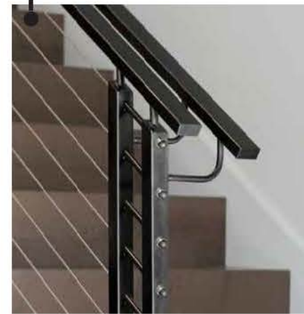
Painted steel flange rails w/ SST cables
