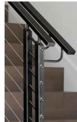
Painted Rails w/ SS cables
