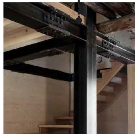
Painted steel structure
