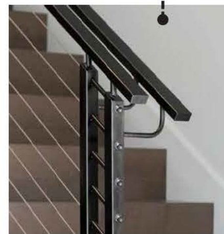
Painted steel fl t-bar rails w/ SST cables
