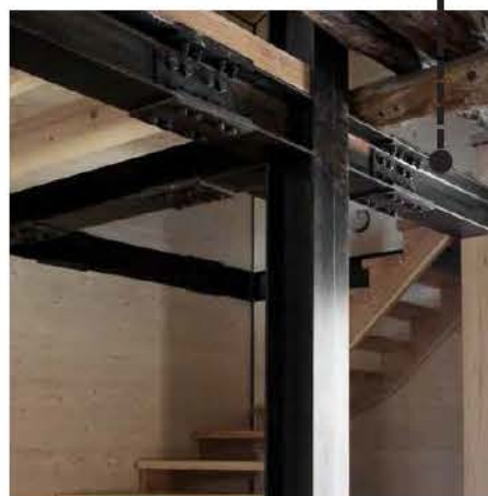
Painted steel structure
