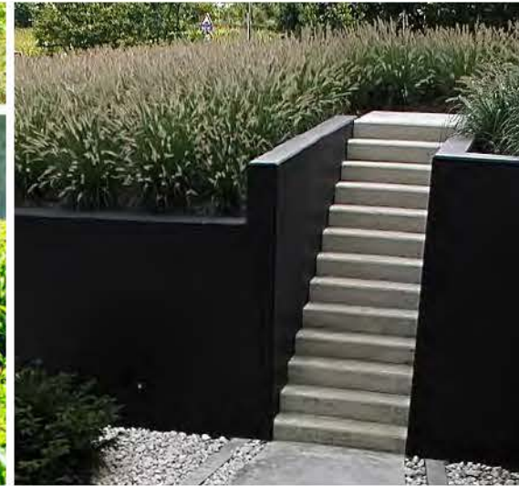
Painted Steel Planter Walls
