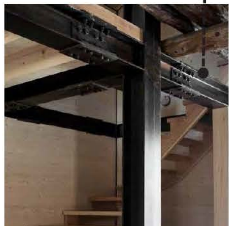
Painted steel structure
