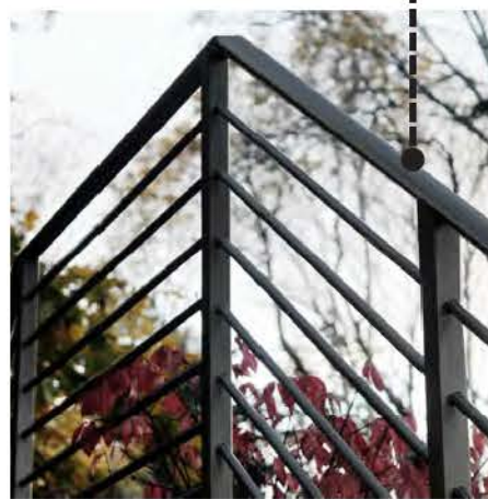
Painted steel rails w/ horiz. rods
