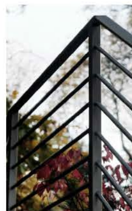
Painted steel rails w/ horiz. rods
