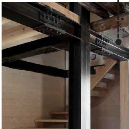
Painted steel structure
