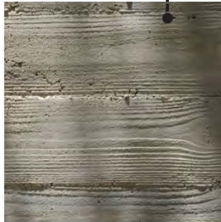
Board - Formed Concrete
