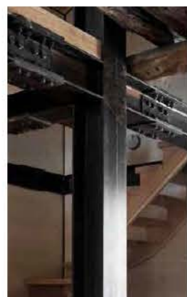
Painted steel structure
