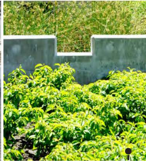
Concrete Planter Walls
