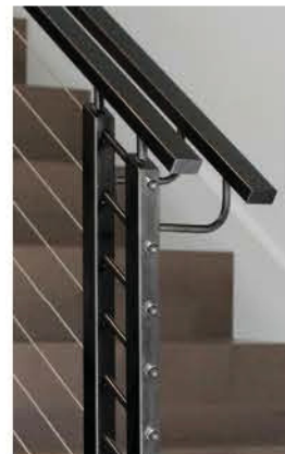
Painted steel rails w/ SST cables
