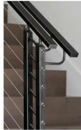
Painted steel rails w/ SST cables
