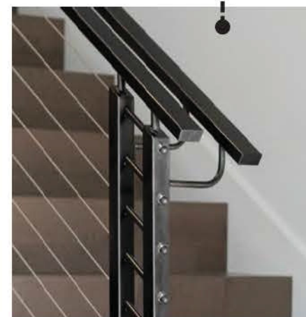
Painted steel flange rails w/ SST cables
