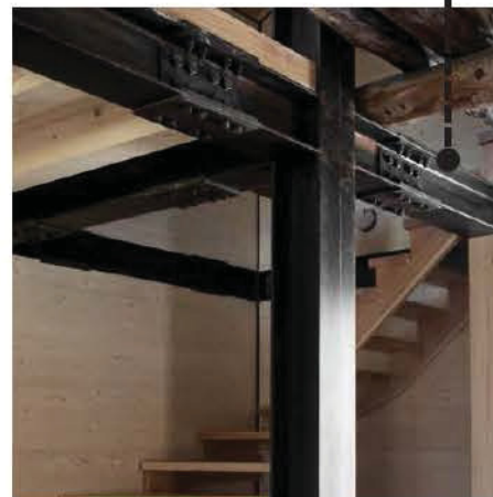
Painted steel structure
