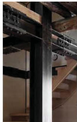
Painted steel structure
