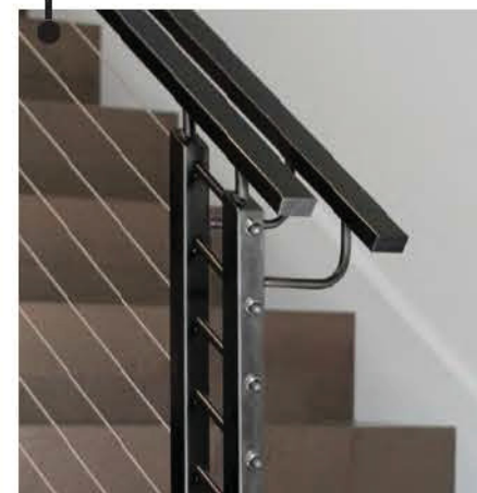
Painted steel flange rails w/ SST cables
