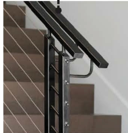
Painted steel flange-t-bar rails w/ SST cables
