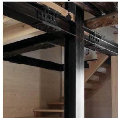
Painted steel structure
