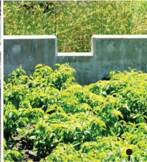
Concrete Planter Walls
