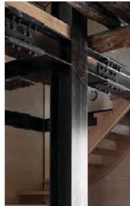
Painted steel structure
