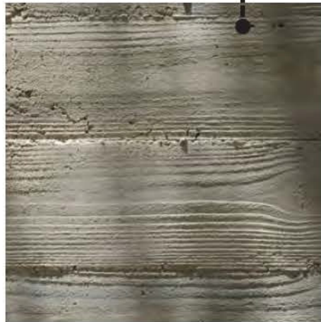
Board - Formed Concrete
