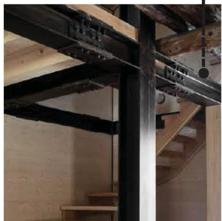
Painted steel structure
