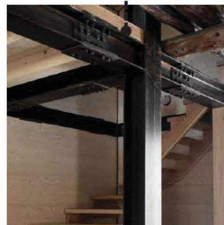
Painted steel structure
