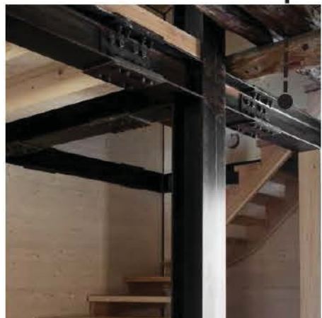
Painted steel structure
