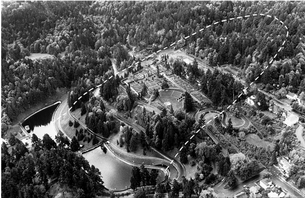
Figure 4. Washington Park Reservoirs landslide. The two reservoirs are at lower left. Perimeter of slide shown by broken white line.
