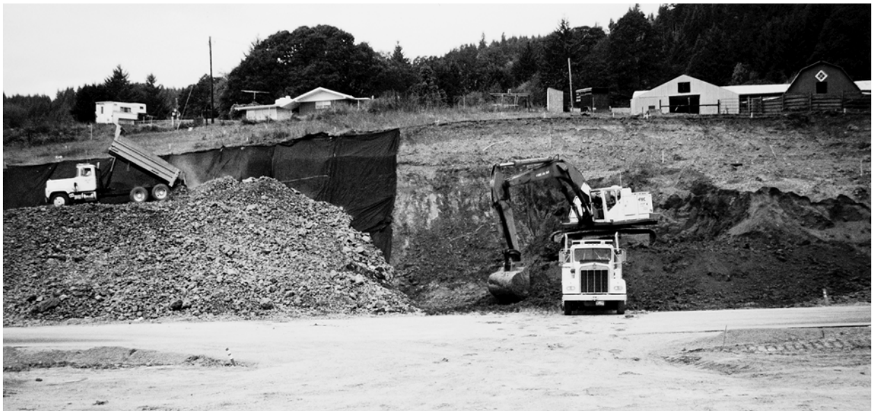
Figure 21. Closely-sequenced construction method being applied at Lorane Road landslide. On right, a backhoe excavates soil and loads spoil into a dump truck. On left, rockfill is being dumped and spread to build a buttress. Filter fabric (dark gray) is laid on the cut slope behind the rockfill.
