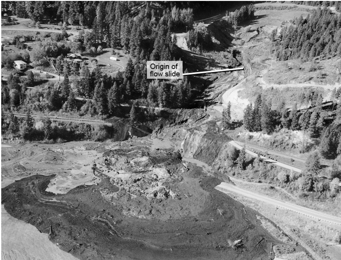
Figure 25. Bonners Ferry landslide. Aftermath of the major flow slide, showing rupture through the railroad embankment and into the flood plain (in foreground). (Photo: David Kramer)
