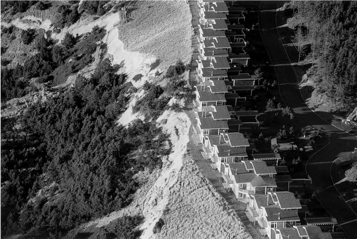
Figure 2. The Capes landslide. Headscarp close to houses on bluff.
