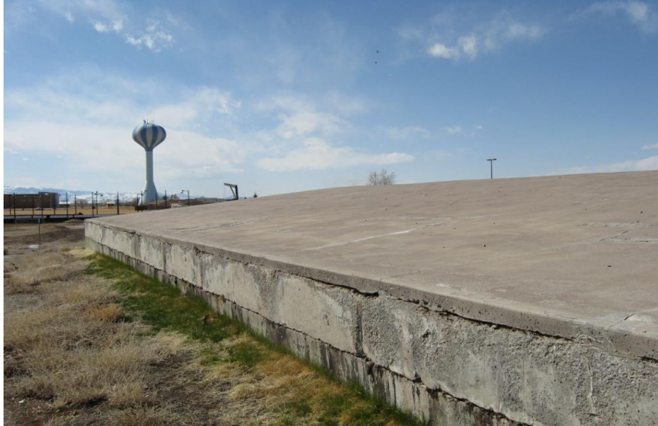
Covered Alamosa, Colorado reservoir where Salmonella bacteria from prolonged bird roosting exposures were not visible or detected, causing illness and death
