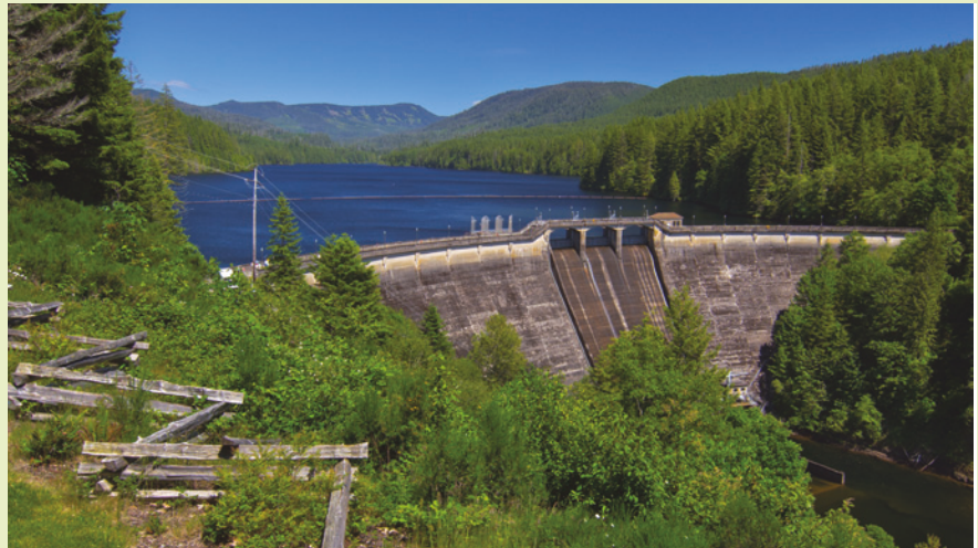
Dam 1 in the Bull Run watershed
