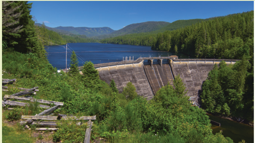
Dam 1 in the Bull Run watershed
