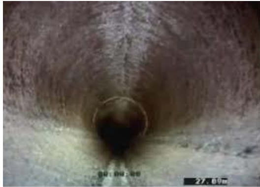
Scheduled routine flushing of system can remove microorganisms. Above is an example of properly maintained water pipe that has been routinely flushed.
