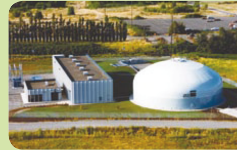
Groundwater Pump Station
