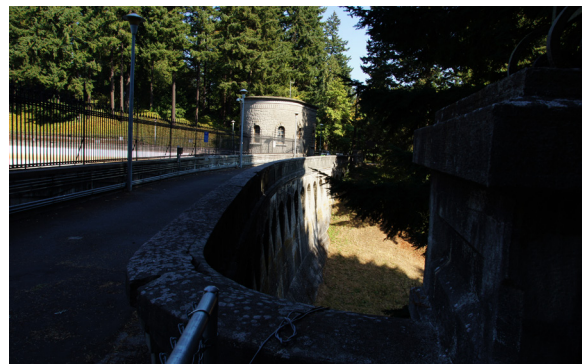
Dam 3, current conditions
