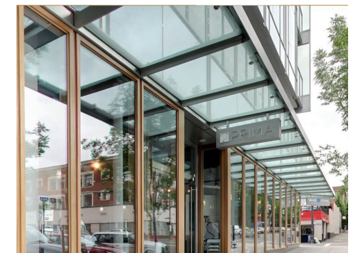
REPRESENTATIVE IMAGE OF STEEL GLASS CANOPY
