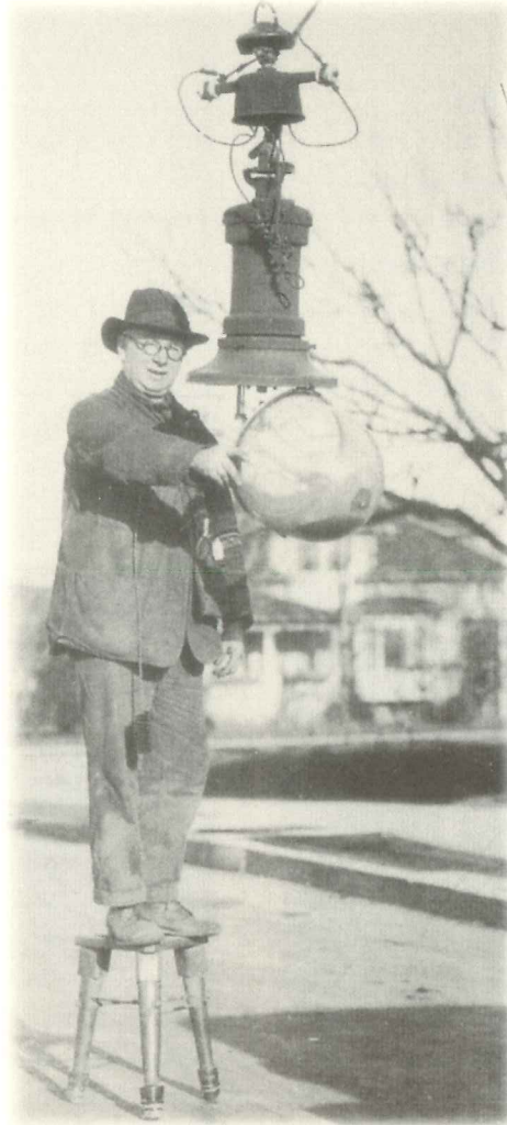
Joseph Poffenberger keeping the arc light trimmed in Portland's Woodlawn district in 1927. A PGE employee from 1899 to 1931, he was responsible for all 953 lamps north of Prescott. Arc trimmers also cleaned the globes and inspected and replaced the suspension cables.
