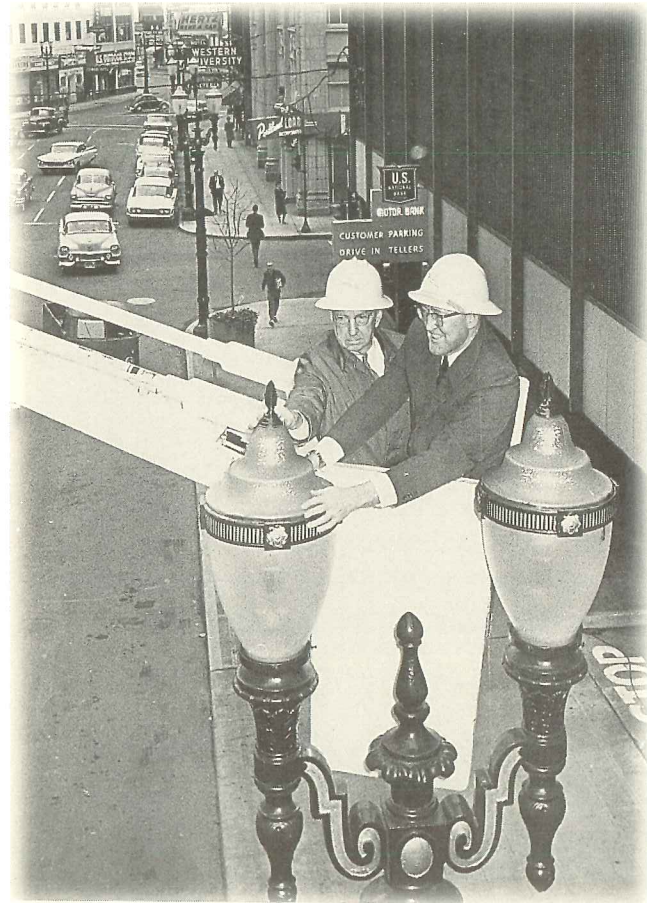
Leonard Bacon photo, The Oregonian Commissioner Ormond R. Bean (left) and Hilbert Johnson, Portland General Electric Co. Vice President (right) converting Portland street light to mercury vapor from incandescent.
