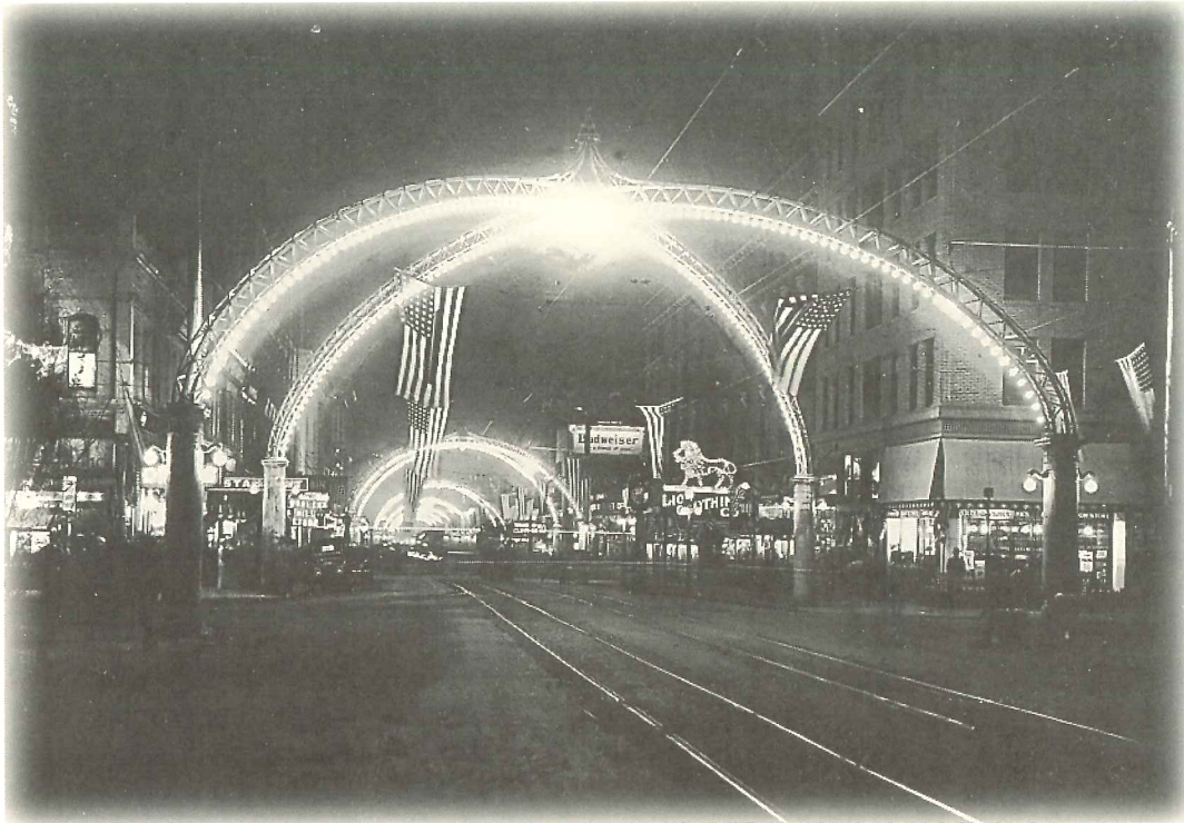
Third Street Arches at night looking North on 3rd and Morrison.
