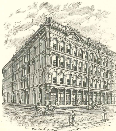
BLAGEN BUILDING. (Erected 1889.) 1190
