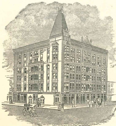
PERKINS BUILDING. (Now building.)
