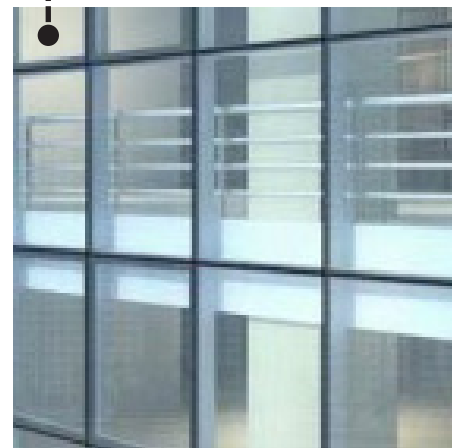
Structural silicone glazed storefront
