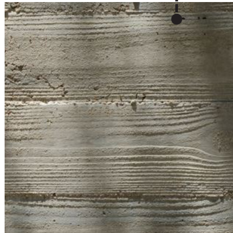
Board - Formed Concrete
