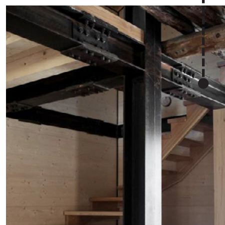
Painted steel structure
