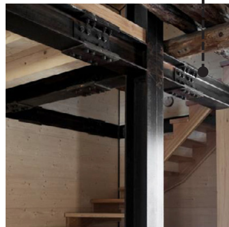
Painted steel structure
