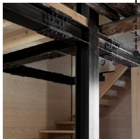
Painted steel structure
