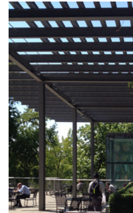
Painted Steel Trellis
