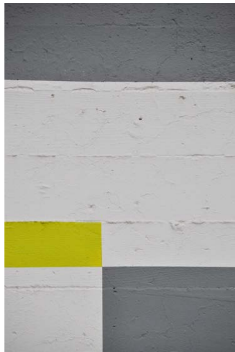
Existing PNCA painted concrete
