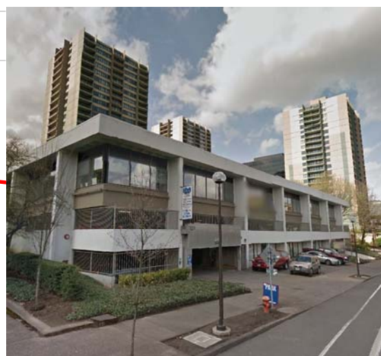
1 st & Harrison, Harrison Towers beyond
