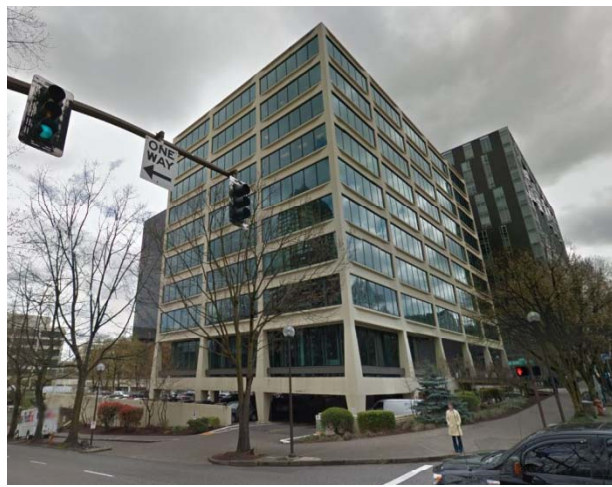
Portland State University, Market Center Building, 4 th & Market
