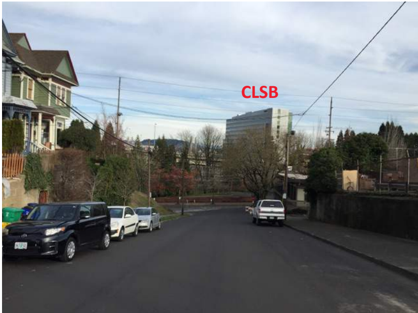
View from Arthur Street at SW Water Ave
