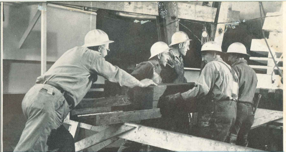
A2004-002, 2244 A2004-002, 2250 Old and new skills of all kinds joined hands to produce ships. At left, a woman painter does her bit on a girder. Above, a crew of workers operate the "ram" which shifts the weight of the vessel before launching. Below, electricians install a switchboard.
