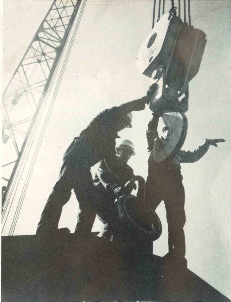
Riggers signal "take it easy" as a huge whirley boom is lowered to hook on to another section for the ways.
