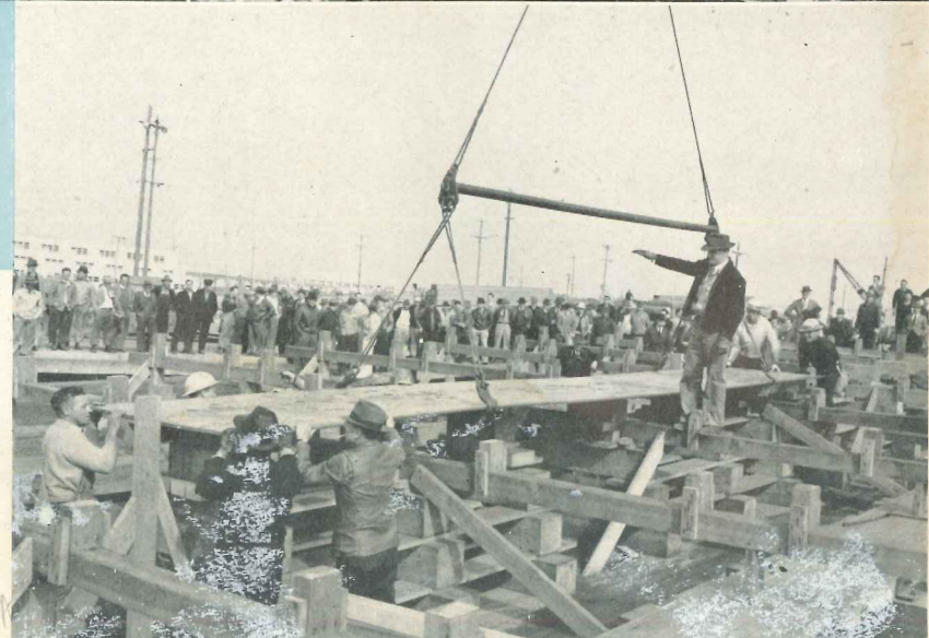
A2004-002, 2262 Scan scan A2004-002, 2203 Shipbuilding in prefabricated style involved many "big lifts" such as these shown here. Above, a huge deckhouse section is carried to the ways by two gantry cranes to be lowered into place on a tanker hull. Above, right, in another two-crane lift, the forward flight deck section is placed on a Vancouver carrier. Lower, right, one of the first Liberty keels being laid at Oregon Ship. Left, finishing touches are put on a Liberty just before launching.
