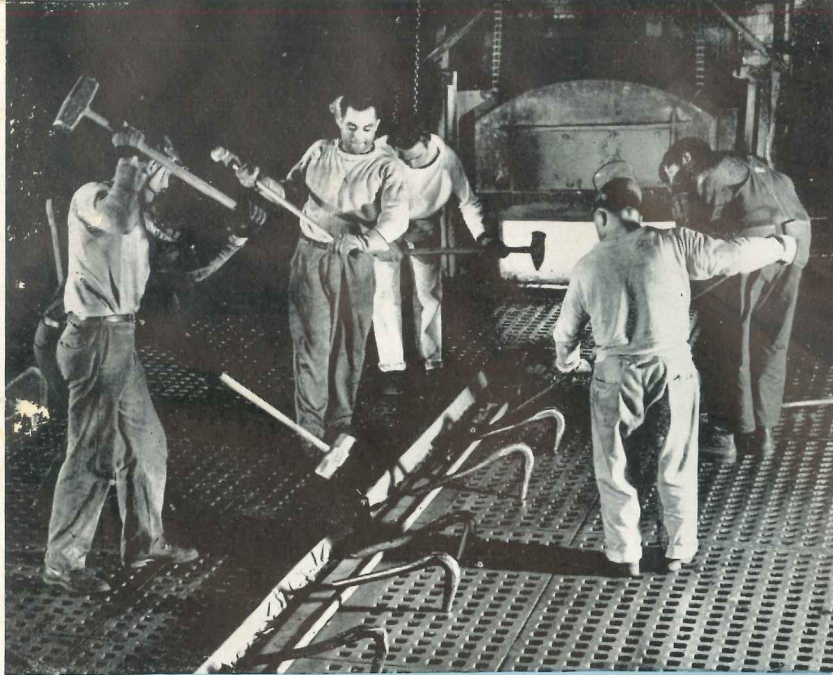
On the "Slab" in the Plate Shop heavy girders are bent into proper shapes. Slab crews are proud of the toughness of their jobs. Lower—A group of employees welding in the Pipe Shop.
