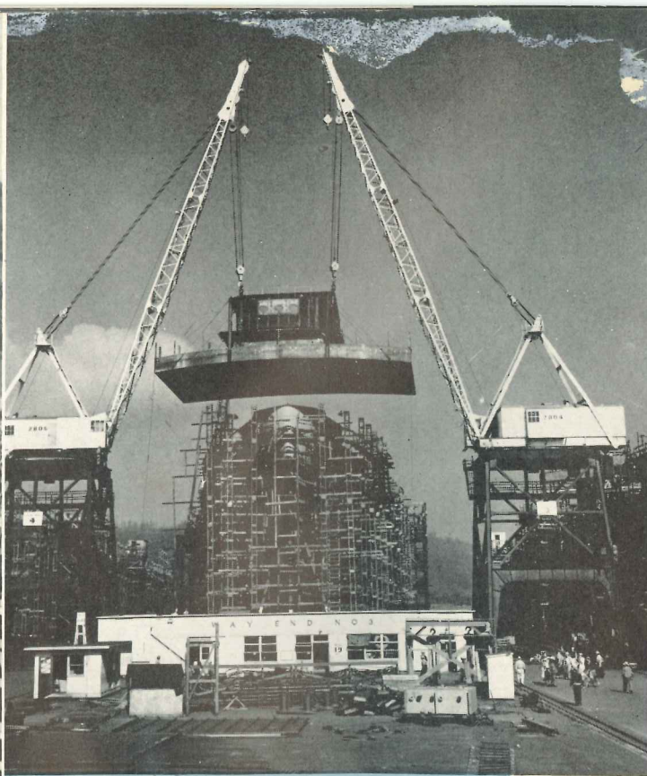
A2004-002, 2262 Scan scan A2004-002, 2203 Shipbuilding in prefabricated style involved many "big lifts" such as these shown here. Above, a huge deckhouse section is carried to the ways by two gantry cranes to be lowered into place on a tanker hull. Above, right, in another two-crane lift, the forward flight deck section is placed on a Vancouver carrier. Lower, right, one of the first Liberty keels being laid at Oregon Ship. Left, finishing touches are put on a Liberty just before launching.
