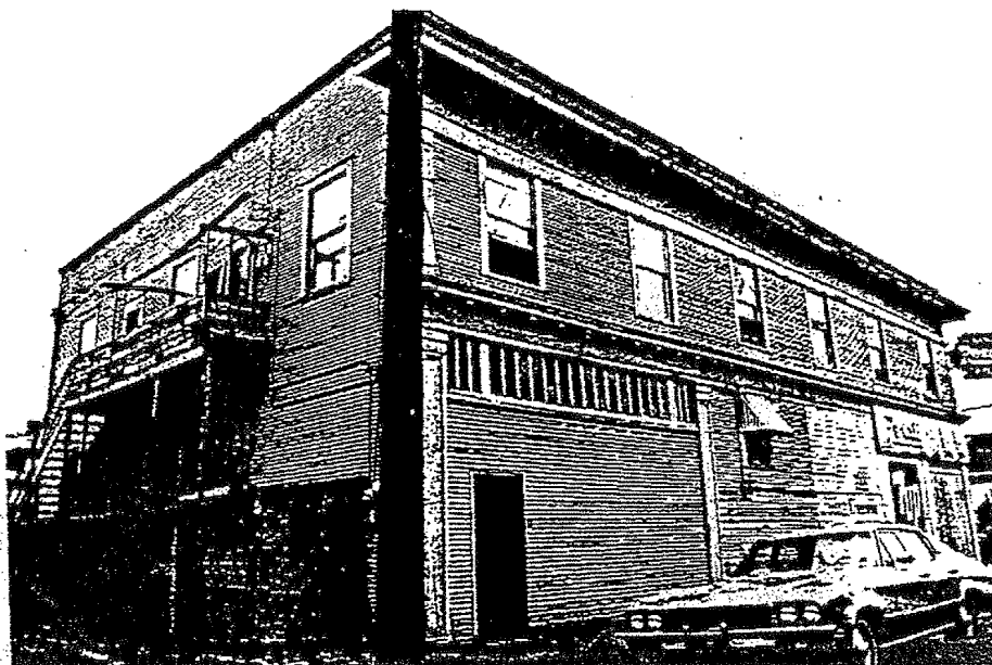
2403 NE Alberta Street. Streetcar Era Commercial Apartment House, 1909.
