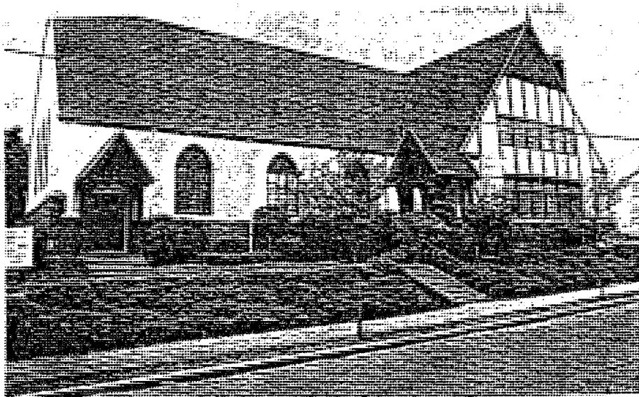
4635 NE 9th Avenue. Highland Congregational Church, 1926.
