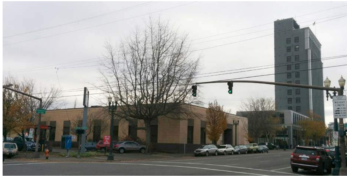
APPROACH ON SE MORRISON ST
