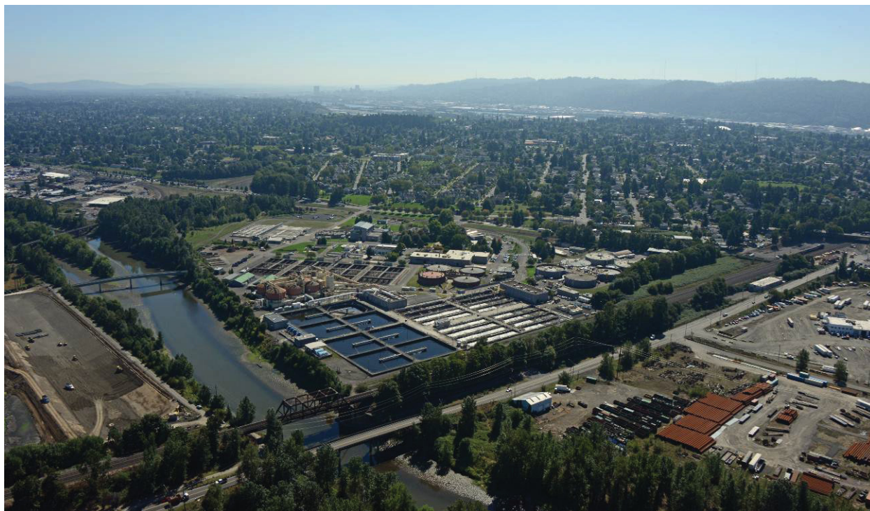
Columbia Boulevard Wastewater Treatment Plant
