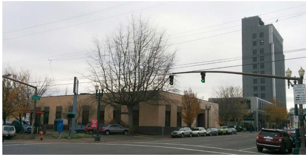
APPROACH ON SE MORRISON ST
