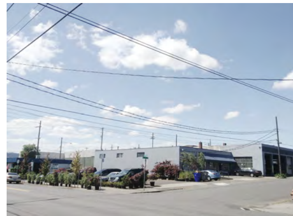
Intersection of 9th and Stark
