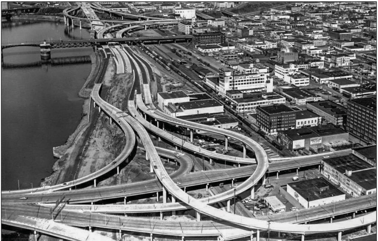
Construction of I-5 and the Morrison Bridge Eastbank Interchange in 1963.
