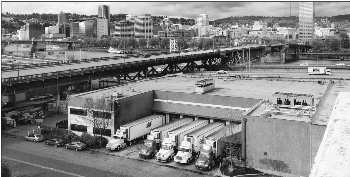
Trucks loading and unloading at the Pacific Coast Fruit location on 2nd Ave adjacent to a mixed use tower being constructed across the street and the Eastside Exchange industrial office building.
