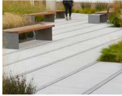
CONCRETE PAVERS/WOOD BENCH
