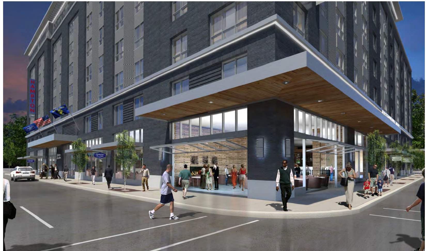
NW 9TH AVE & NW EVERETT ST
