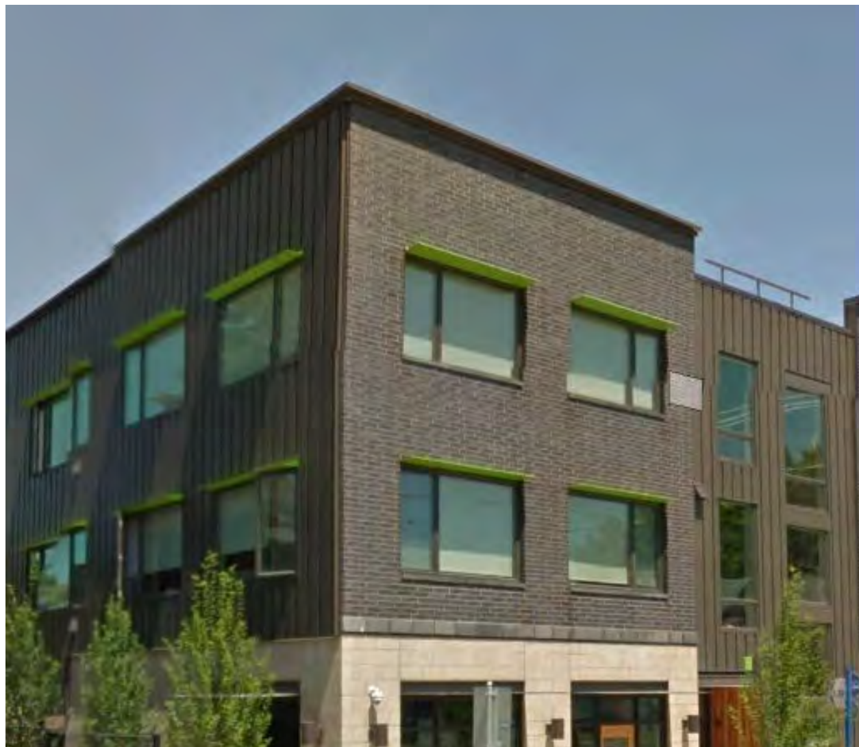
Mutual Materials Coal Creek installation photo.
