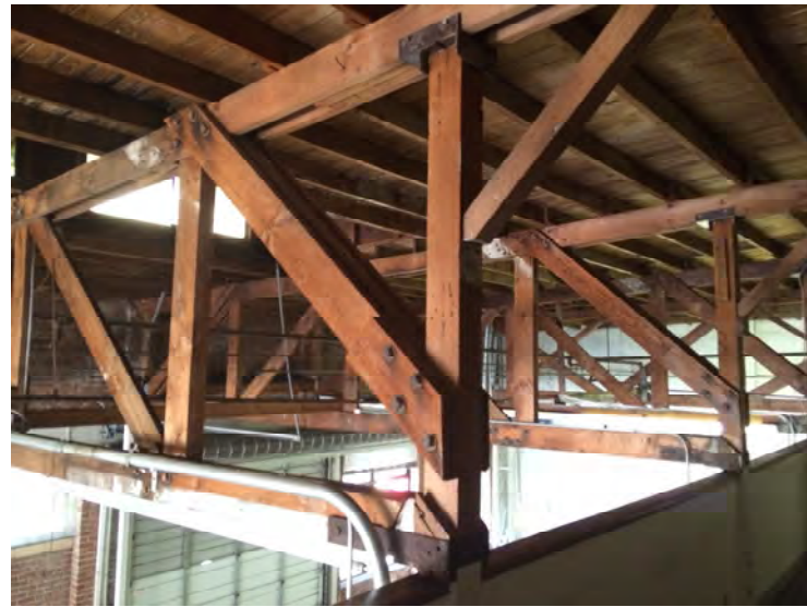
Existing Trusses—821 NW Everett St
