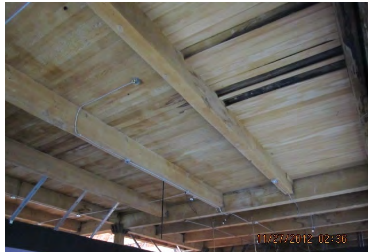
Existing Floor Boards 338 NW 9th Ave
