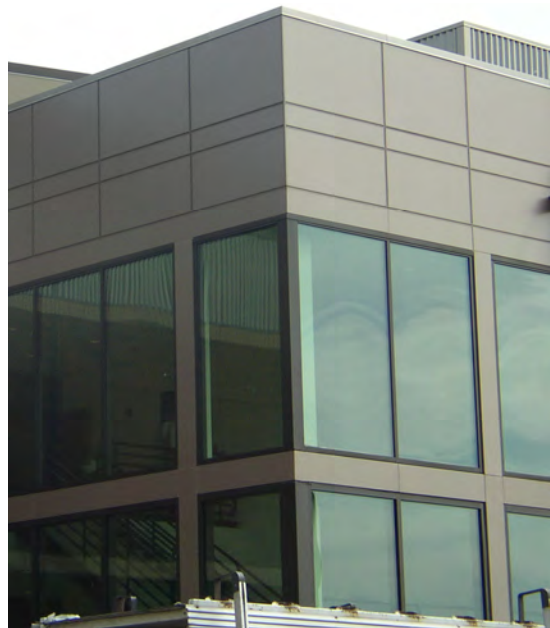
Clear Anodized Metal Panel Installation Images
