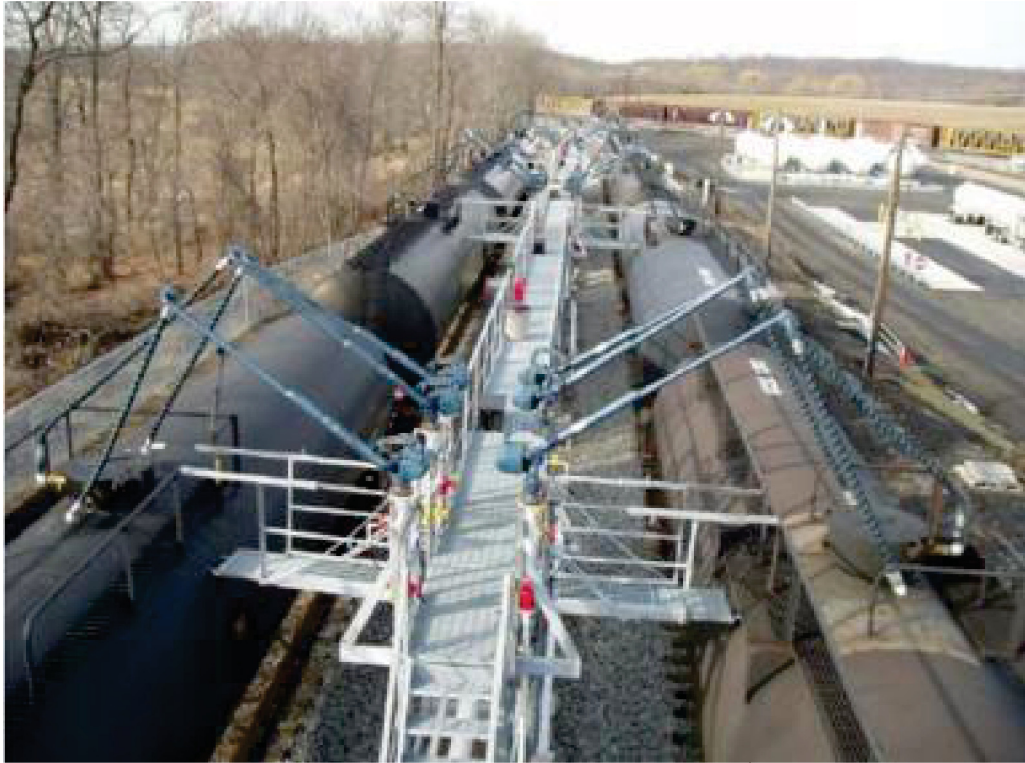
Figure I-20: Rail Car Offloading Arrangement (Ref. 3)
