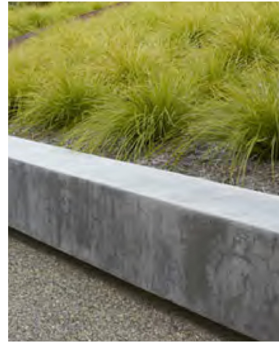
CONCRETE SEAT WALL
