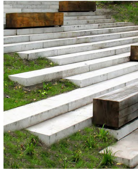
CONCRETE SITE STEPS
