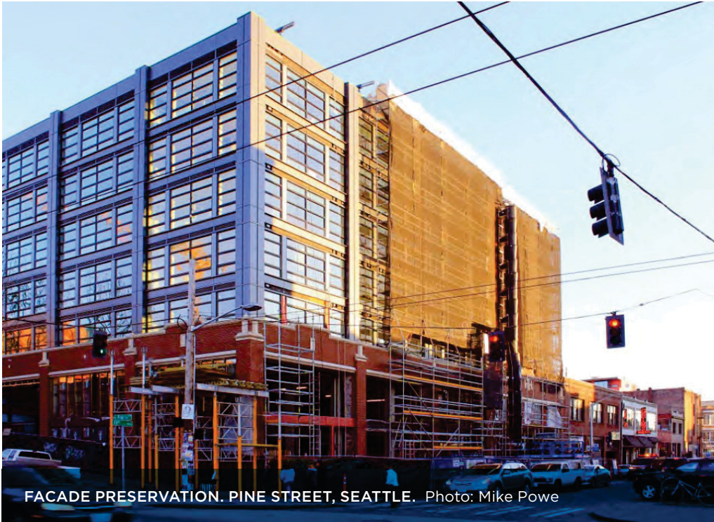
The historic facade from the Sunset Electric building (1916) on Pine Street stands below a nearly-completed 89-unit apartment building.
