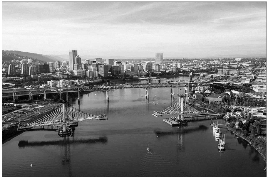
The Tilikum Crossing Bridge under construction, late 2013
