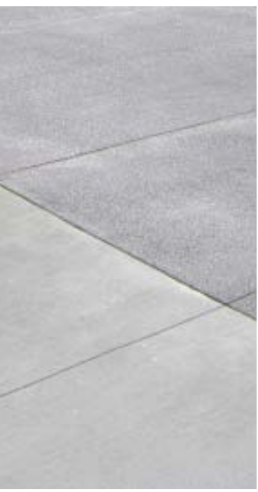
enhanced concrete paving poured-in-place concrete paving with integral color and decorative aggregate with acid etch or light sandblast finish application.
