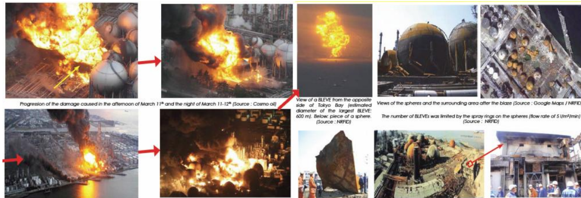
Figure 6: Cosmo Oil’s LPG terminal in Tokyo Bay is built on harbor fill consisting mainly of water-saturated sandy alluvial soils (LPG is a mixture of gases, including propane). This high seismic risk location and facility has many similarities to the site of Portland’s proposed propane export terminal. On March 11, 2011, an earthquake similar in magnitude to Portland’s expected “big one” caused structural failure and tank collapse due to soil liquefaction. A lethal domino cascade ensued, which over a period of three hours, included a large vapor cloud explosion, and five BLEVEs the largest of which had a fireball diameter of almost 2,000 feet. All told, seventeen LPG tanks were destroyed. Damage included thermal radiation, overpressure blast, and rocketing tank fragments and other debris. Cleanup took two years.
