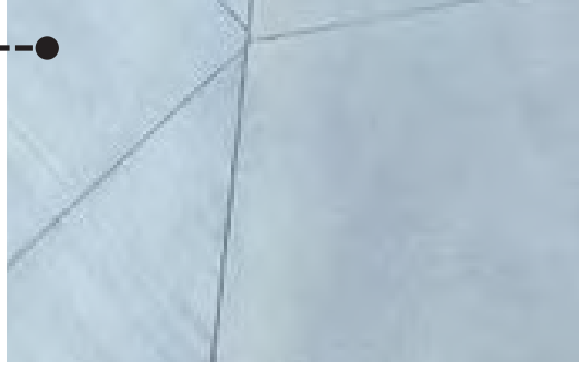
Sawcut Concrete Score Pattern
