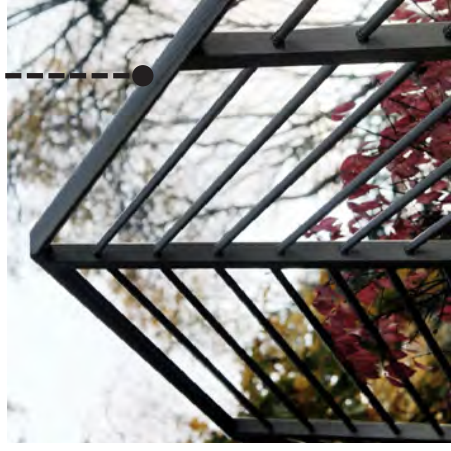
Painted steel rails w/ horiz. rods
