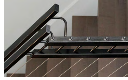
Painted Rails w/ SS cables
