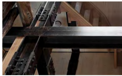
Painted steel structure
