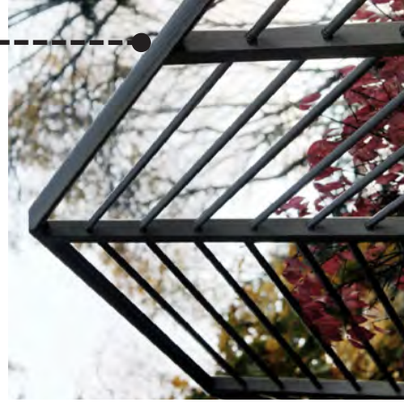
Painted steel rails w/ horiz. rods
