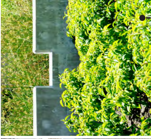
Concrete Planter Walls
