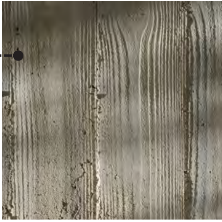
Board - Formed Concrete
