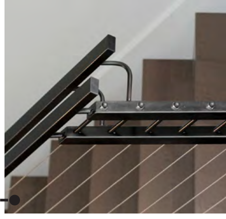
Painted steel flat-bar rails w/ SST cables
