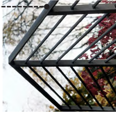
Painted steel rails w/ horiz. rods
