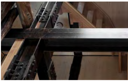
Painted steel structure
