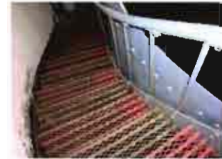
Curved iron stairway, interior Gatehouse 1
