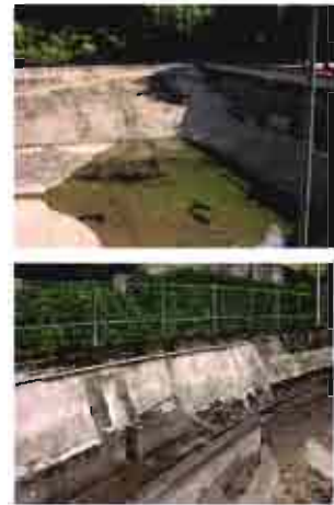
Reservoir Structure, Reservoir 1
