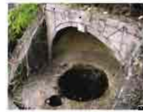
Reservoir 1 Fountain Structure
