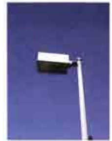
Non-historic light posts, Reservoir 5
