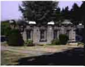
Hypochlorite Building (Weir House) Gatehouse 5
