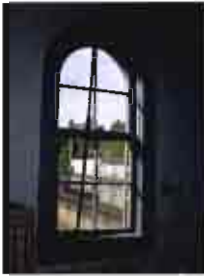
Typical Window, Gatehouse 5
