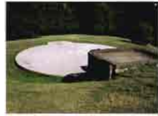
Reservoir 7 Underground Tank Structure
