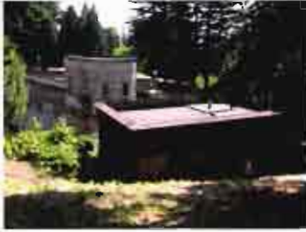
Reservoir 1 Weir Building
