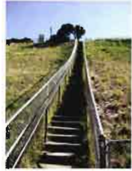
Stairway, Reservoir 5 to Reservoir 6
