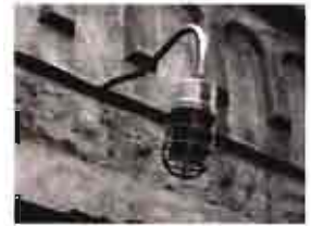
Historic exterior light over door
