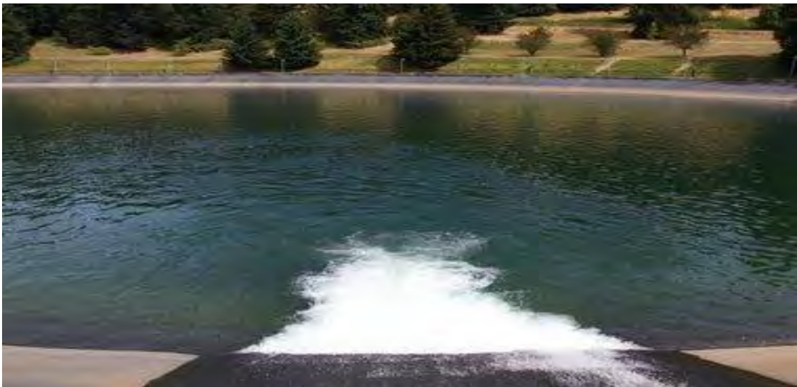
Mt. Tabor Reservoir 5. Open reservoir drinking water inlet: waterfall agitating action aerates water providing oxygen, promotes water movement, while removing unwanted gases. Open reservoir sunlight also provides a public health barrier, using a natural, sustainable, gravity fed carbon-free process delivering safe and healthy water.
