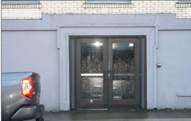
Figure 23 (left) and 24 (right): Lower Third Covered with New Cement; New Glass Doors; Infilled Street Windows
