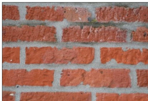
Figures 21 (left) and 22 (right). Sandblasted Brick with Cement Mortar
