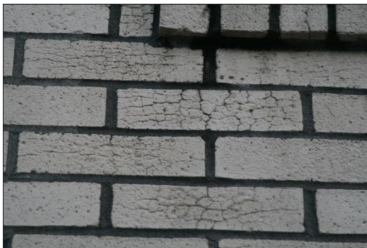
Figures 21 (left) and 22 (right). Sandblasted Brick with Cement Mortar
