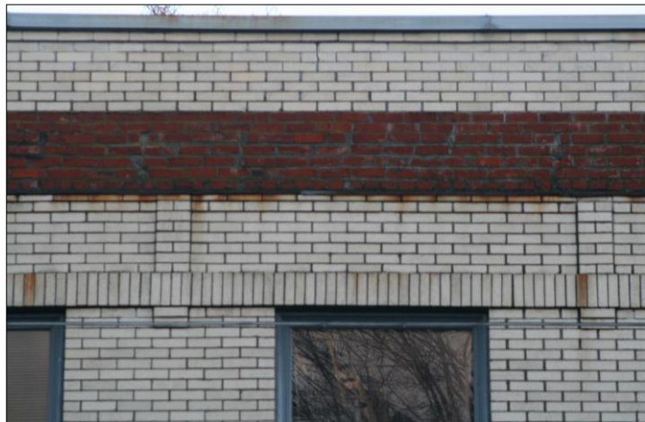
Figure 26. Cornice Removed
