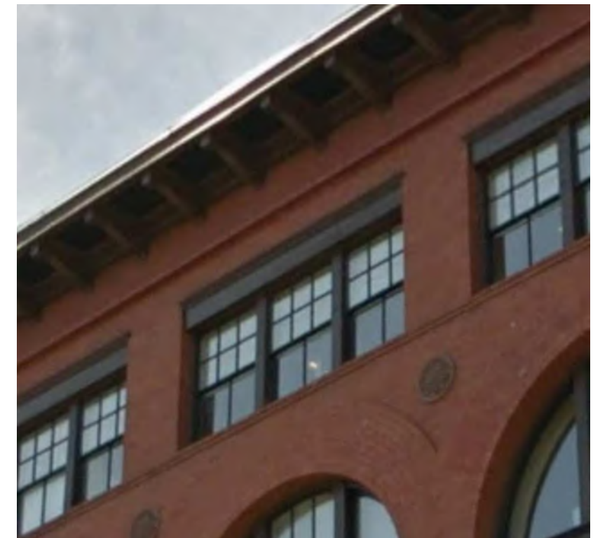
STEEL C-CHANNEL LINTEL ABOVE WINDOWS
