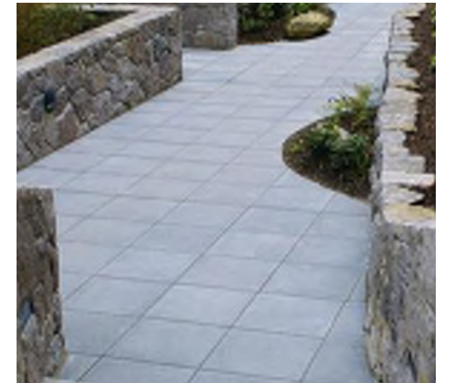
Concrete pedestal pavers
