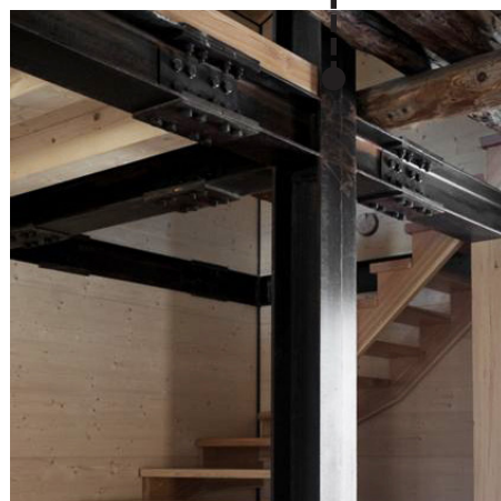
Painted steel structure
