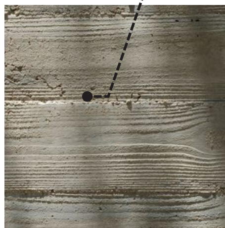
Board - Formed Concrete
