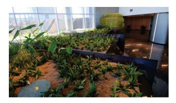
The Living Machine™ is an onsite water treatment system that accepts all wastewater generated by the building's 500 employees and produces water that is reused to flush toilets and supply the cooling towers in the building. The building has demonstrated a 75 percent reduction in water use.
