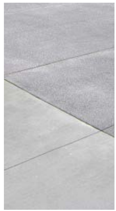
enhanced concrete paving poured-in-place concrete paving with integral color and decorative aggregate with acid etch or light sandblast finish application.
