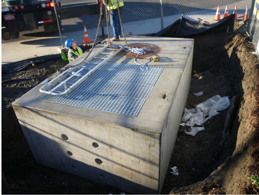
Completed Air Relief Vault for Balch Pipeline
